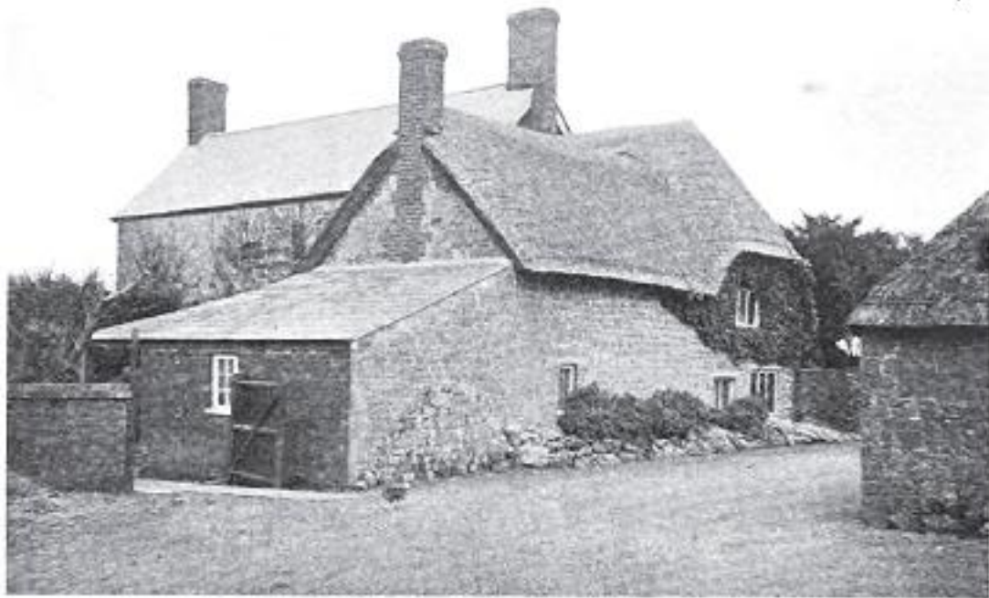
COATE HOUSE FROM THE BACK ; SHOWING THE OLDER PORTION OF THE HOMESTEAD
